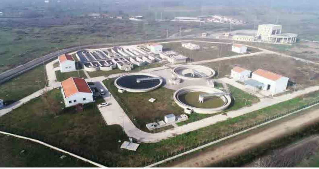
BUSKİ Mustafakemalpaşa Pumping Stations
