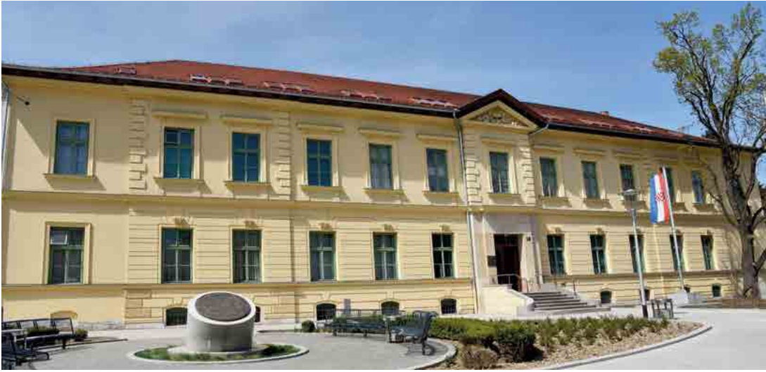
Akfen Construction and Dost Construction won the tender for the Renovation and Reconstruction of Sister of Mercy Hospital (2022)
