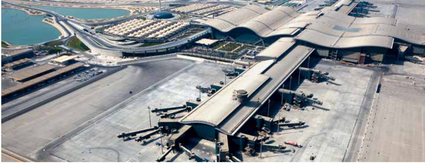
Qatar, Doha International Airport
